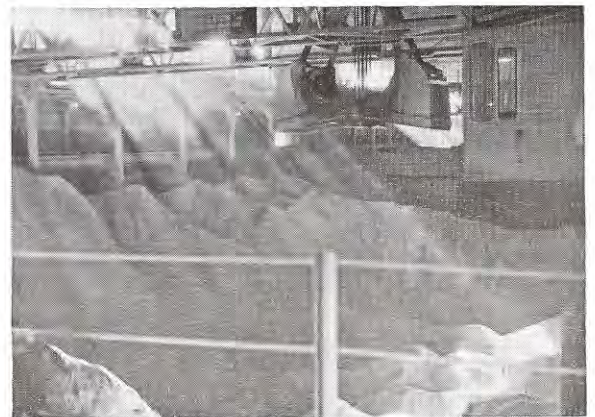
A fantastic photo taken at the Portland Cement Works, Whangarei, of the sun filtering through windows above the storage pit.
